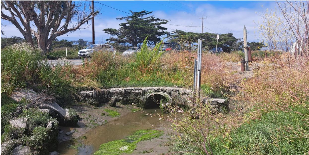
Figure 4 Photo taken from Slough channel, looking NE at the agricultural ditch outlet with existing 42" culvert and headwall.
